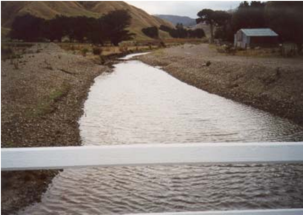
Figure 36: Kakaho Stream, looking upstream from Pauatahanui Road bridge. The banks have been mechanically graded and stripped of vegetation.
