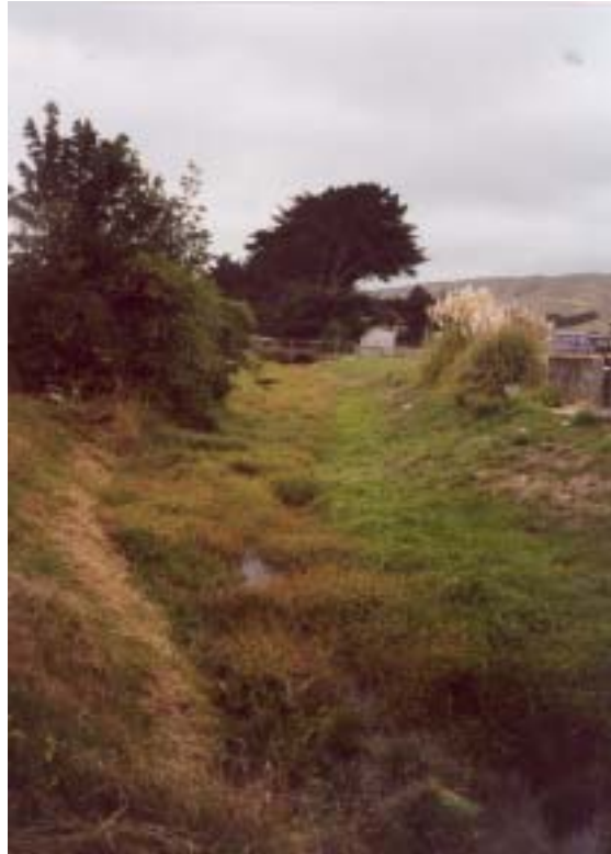
Figure 40: Taupo Stream at the Plimmerton Domain. The channel is partially dewatered, and the banks mown.
