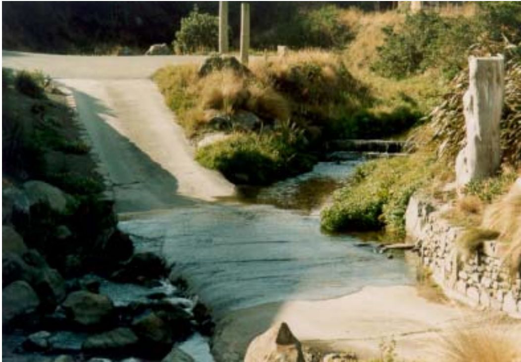
Figure 16: Owhiro Bay Stream. While there was riparian vegetation suitable for spawning, the concrete road ford and weir upstream would inhibit catchment access for inanga.
