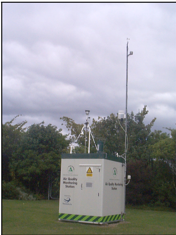
Figure 3.1 Air Quality Monitoring Station
