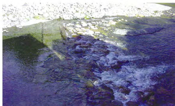
The weir as it is now.
