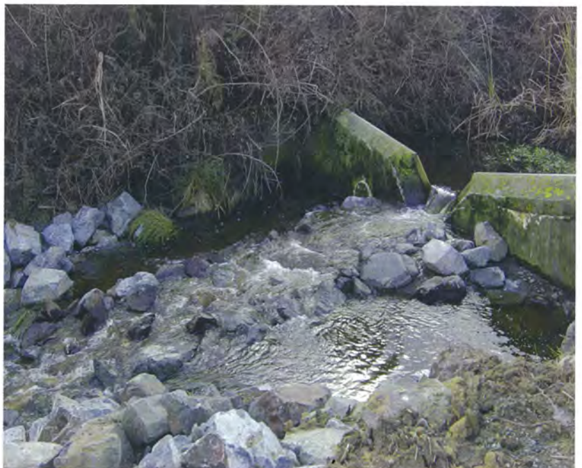
Fish passes like this rock ramp built in the Taupo Stream, below the Taupo Swamp near Plimmerton, help native freshwater fish swim upstream past weirs.
