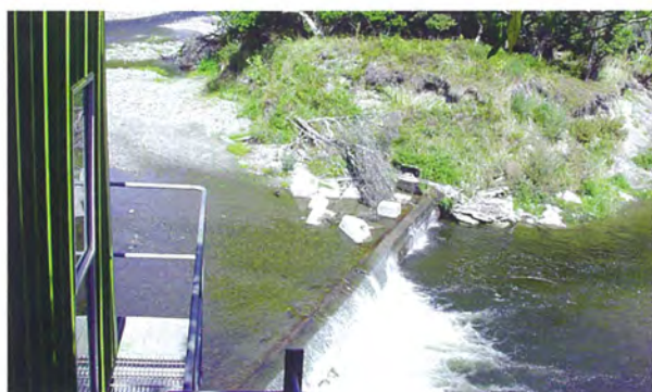
The original Waikanae water supply weir.
