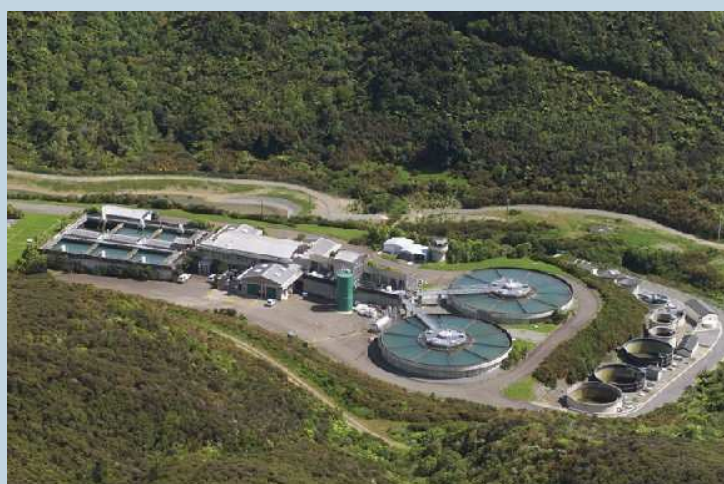
Te Marua Water Treatment Plant
