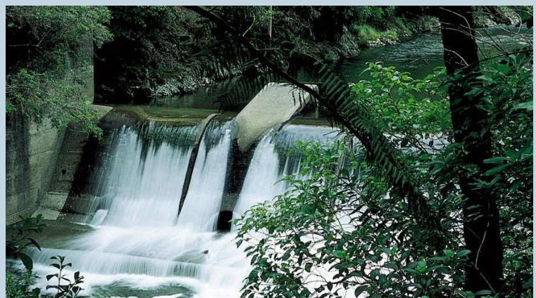
Kaitoke water intake weir
