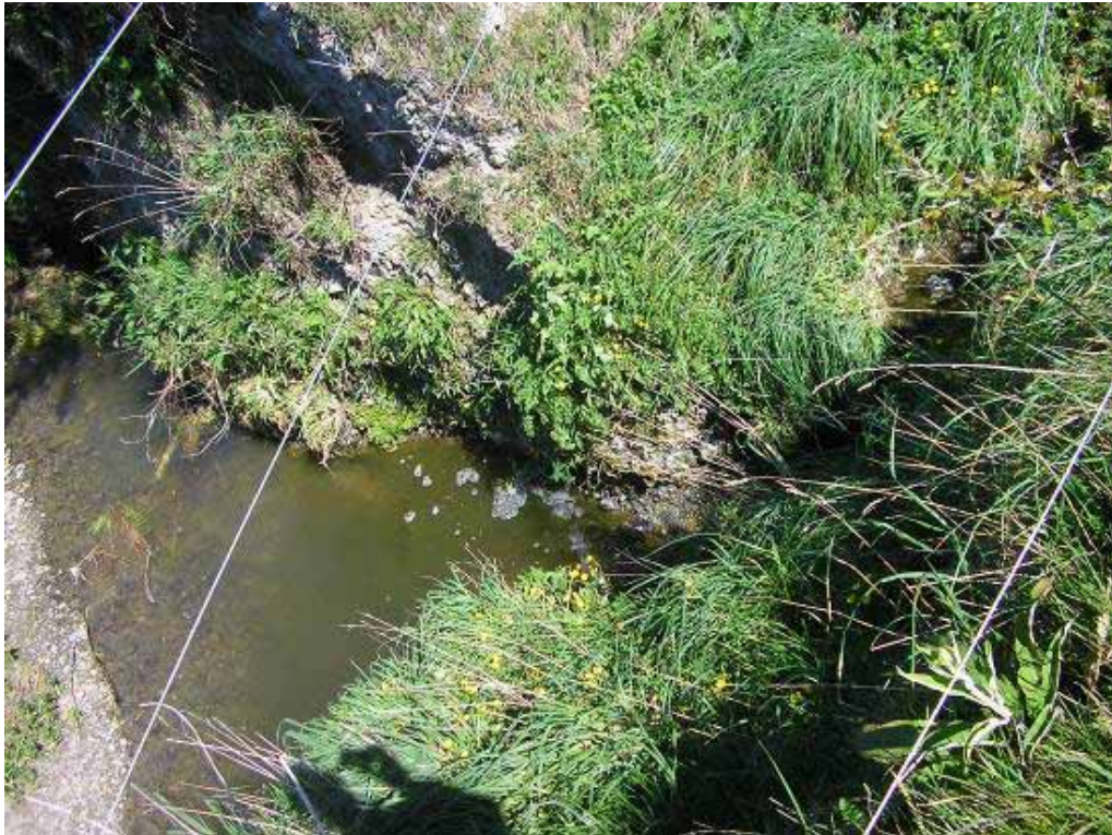
Figure 4.11: Raw dairy shed effluent illegally discharging to a tributary of the Enaki Stream upstream of the rehabilitation area during October 2007.
