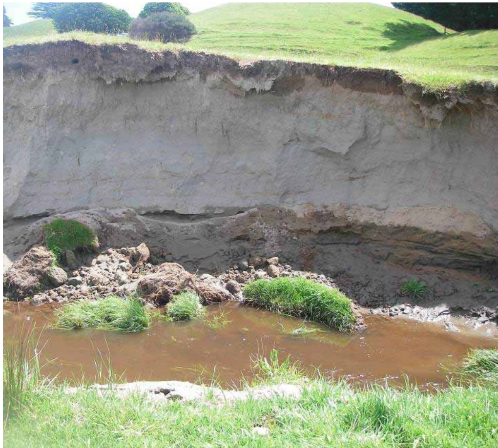
Figure 5.6: Upstream of the rehabilitation area erosion and slumping were common resulting in lower bank stability. Photo taken in 2008.
