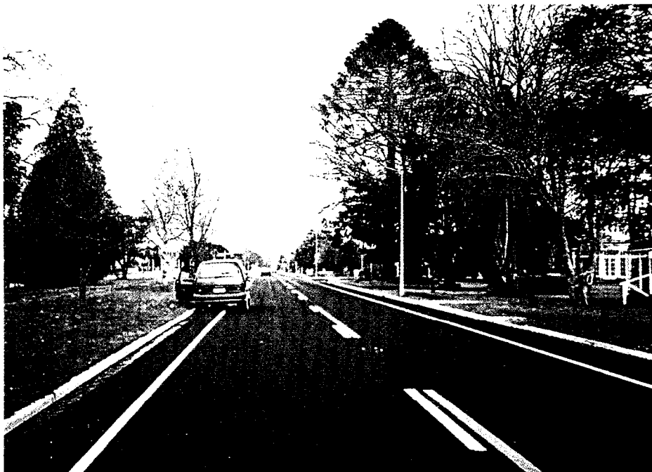
Shoulder width is too narrow for parking, but there are no No Stopping lines to restrict vehicles from parking at the kerbside.
