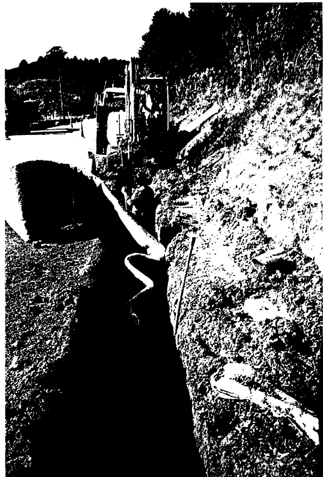
Geosynthetic drain installation Photo: Ground Engineering Ltd
