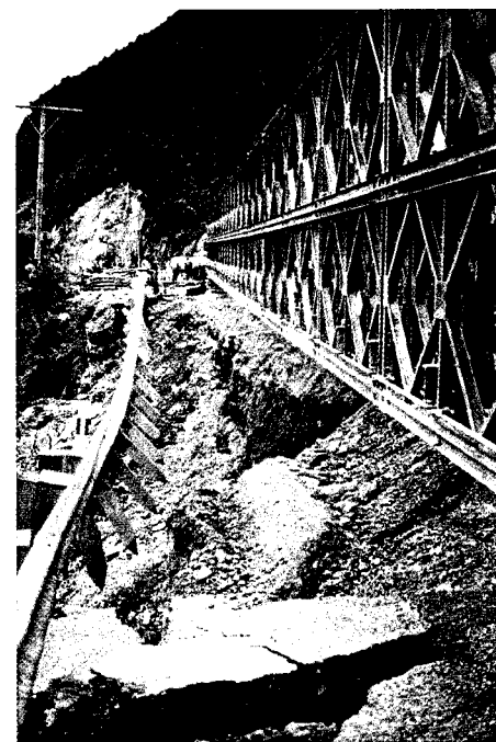
Above: This Bailey bridge on SH6 near Makarora was the only way of repairing the road when it dropped into a gully.
