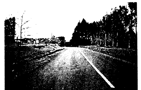
An example of poor application of edge marker posts on a horizontal curve.
