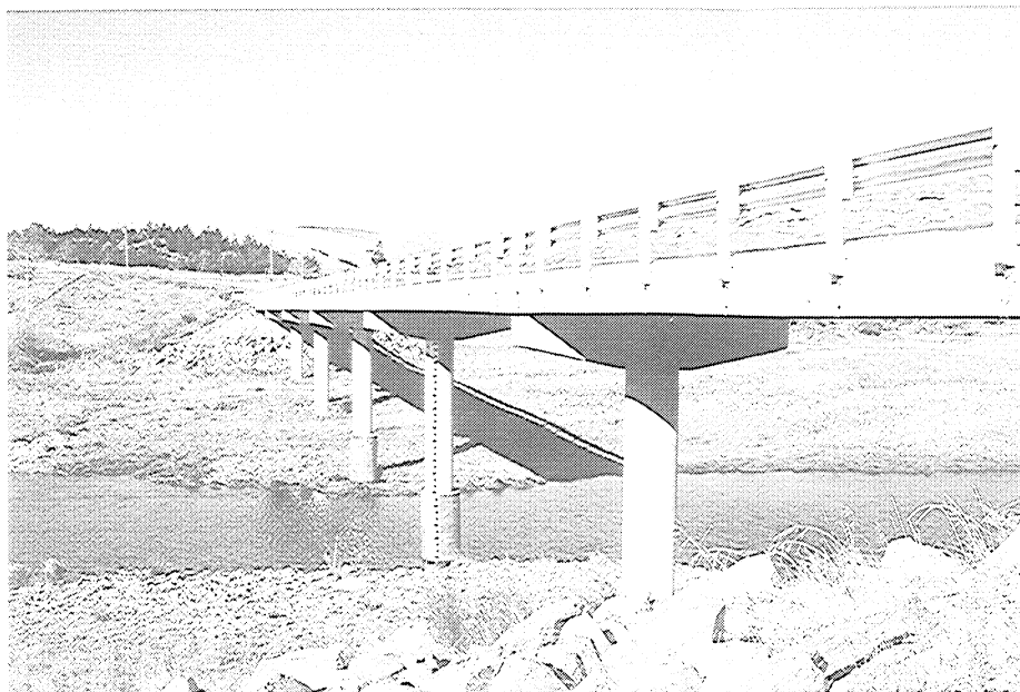
McCulloch's Bridge. Waihou River, Valley Road, south west of Waimate. (From 'Bridge Scour', by Bruce W. Melville and Stephen E. Coleman, Water Resources Publications LLC)
