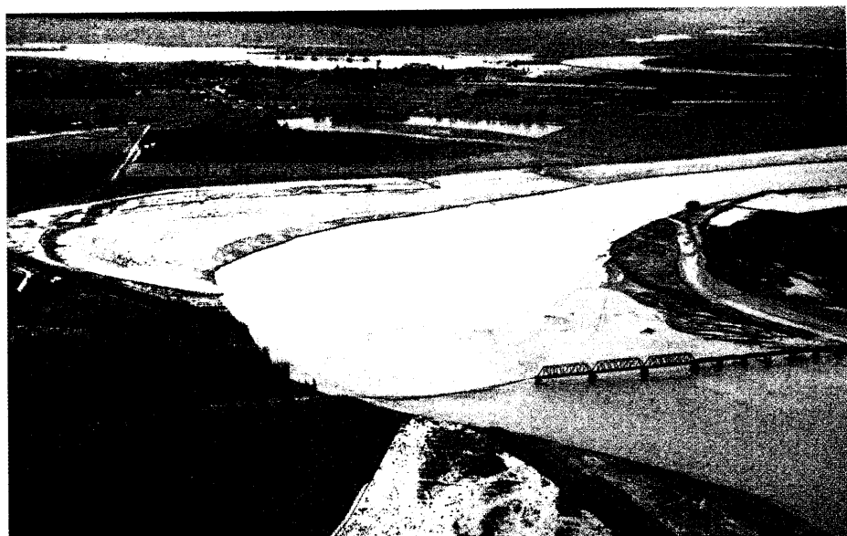
Failure of the railway bridge over the Waipaoa river close to Gisborne during Cyclone Bola.
