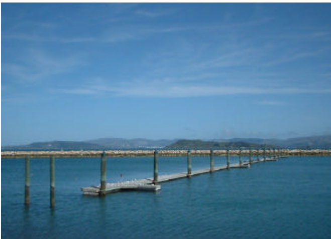
Figure 5 Pile Mooring at Seaview Marina
