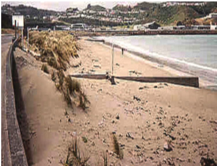
Figure 3 Stormwater Outfall at Lyall Bay, Wellington
