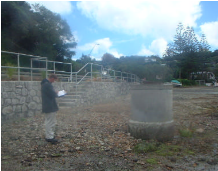
Figure 2 Sewer Inspection Point Located along the Pauatahanui Inlet
