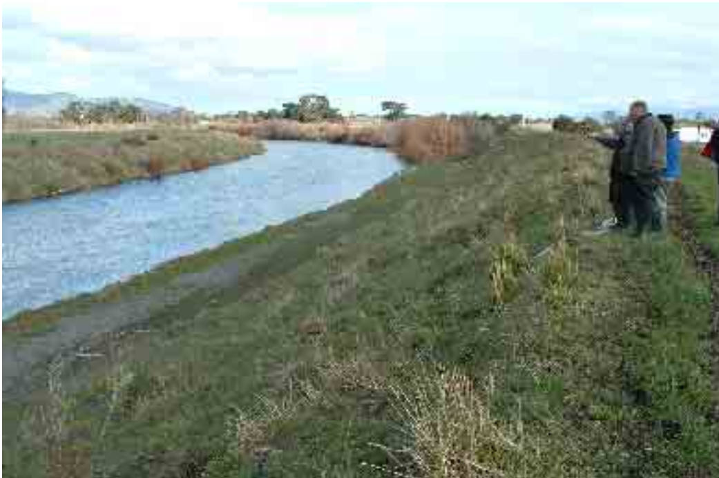
Figure 5: Butcher's stopbank showing silt on the berm and stock damage
