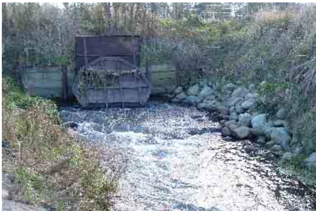
Figure 9: Floodgate from the Muhunua Stream
