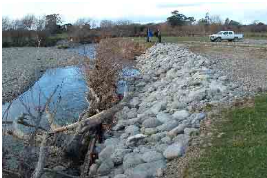
Figure 6: Rail iron deflector fence and newly constructed boulder rip-rap bank protection
