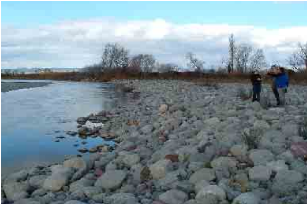
Figure 7: Boulder rip-rap bank protection
