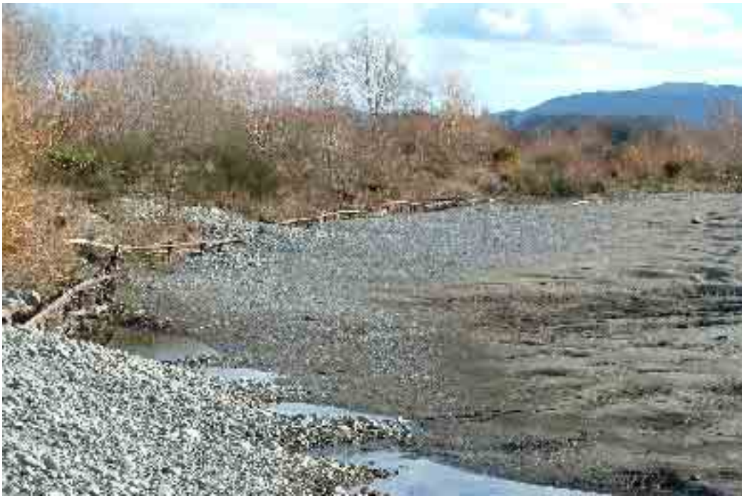
Figure 8: Gravel bank and linear iron training fence
