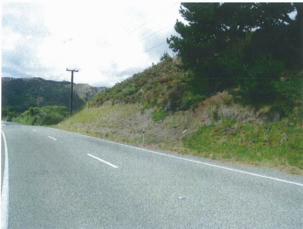
PHOTO: A 37-metre-long retaining wall will be required where this sand dune meets Poplar Ave.
