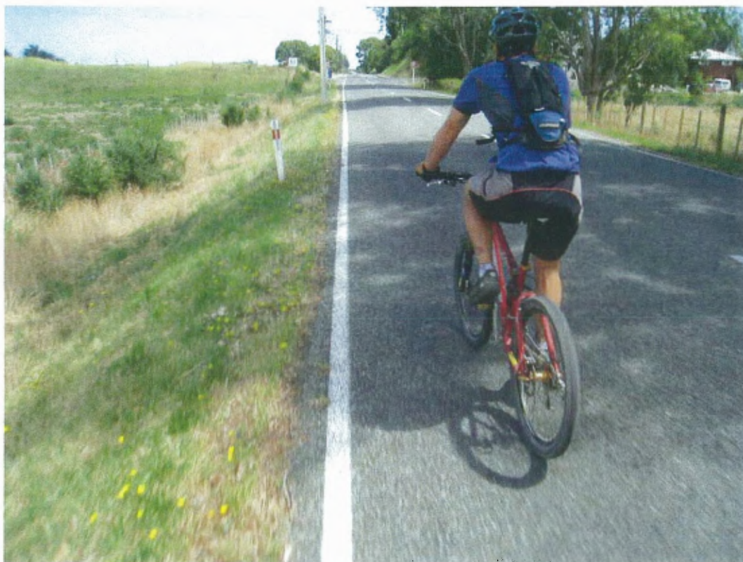
PHOTO: With no shoulder on the side of Poplar Avenue people feel unsafe cycle commuting.
