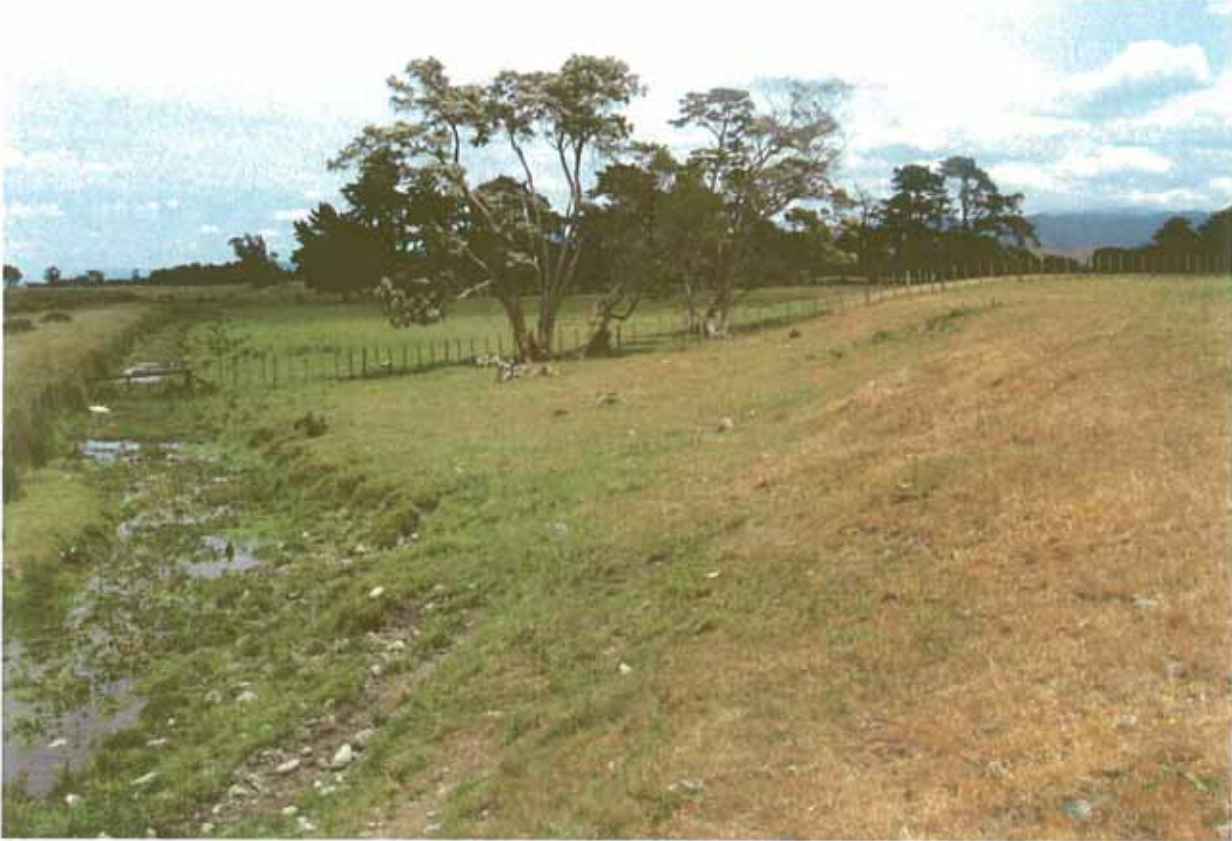
Figure 3: Western Extent of Proposed Extraction Area - Looking West
