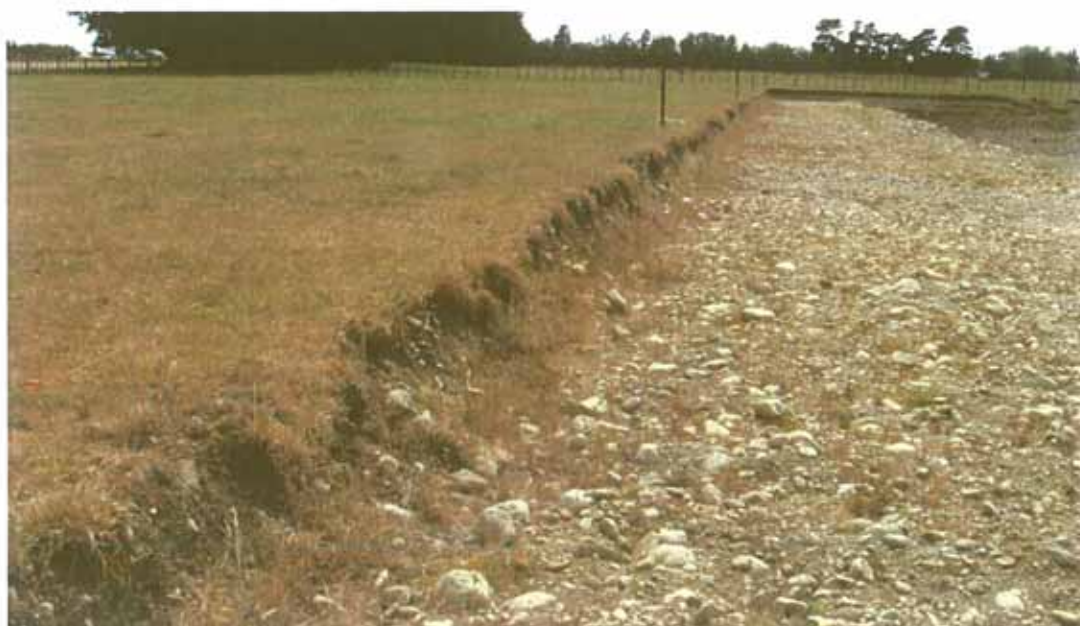
Figure 7: Pre-stripped Northern Section of Existing Excavation - Looking Northeast
