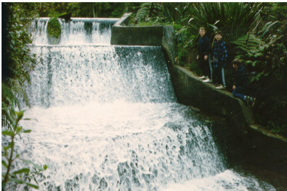
Korokoro Dam (built 1903), Belmont Regional Park (SYD MOORE)
