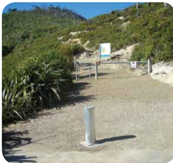
The Ferry Road track was upgraded
