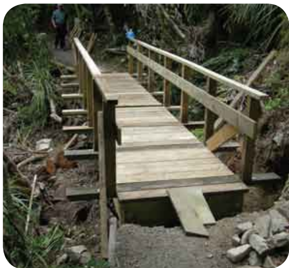
The replacement Mackenzie Track bridge being installed
