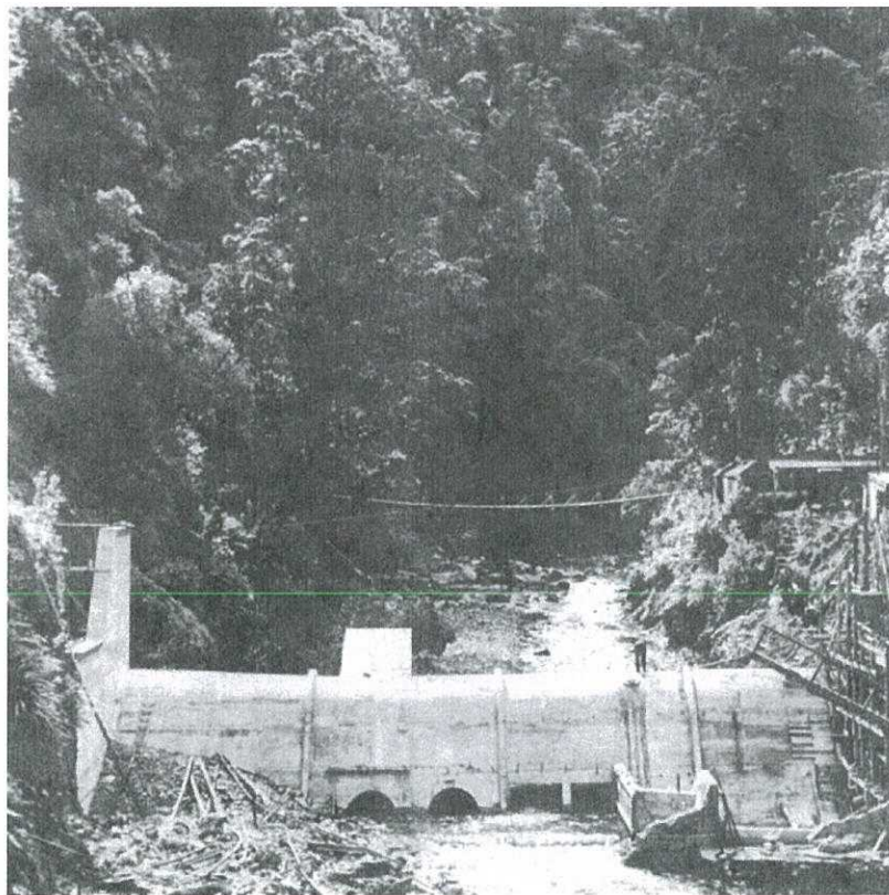
Building the Weir across the Hutt River:
