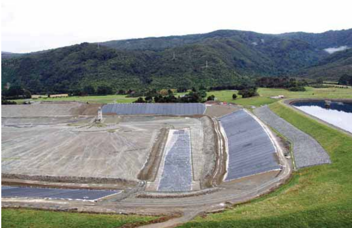
Lining work underway at the Stuart Macaskill Lakes
