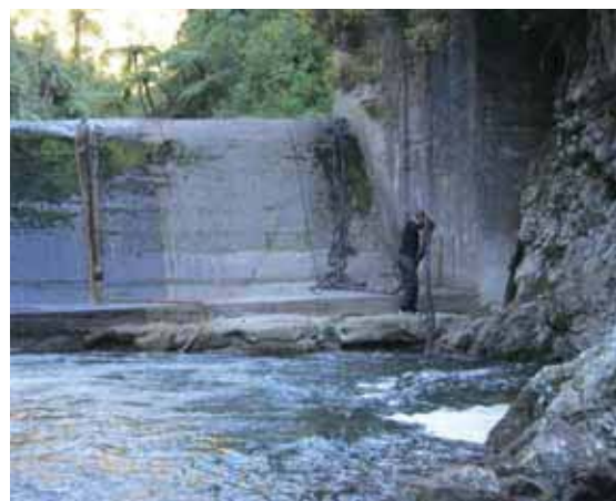
Installing the fish climbing ropes at the Kaitoke Weir
