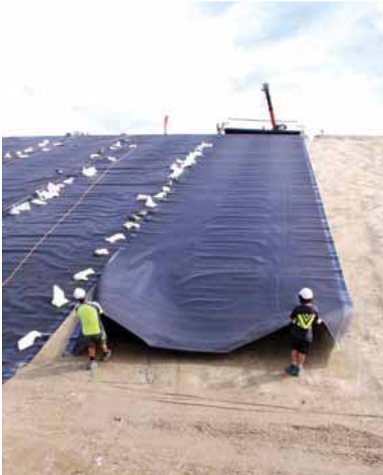
A sheet of plastic liner is pulled into place
