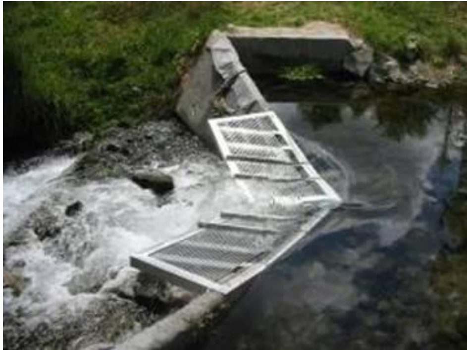
Figure 6. The weir at Hamurana Spring (in the Te Arawa Lakes), utilising an anti-jump grille to exclude trout while allowing passage of native kōaro (Photo: Kristina Thompson).
