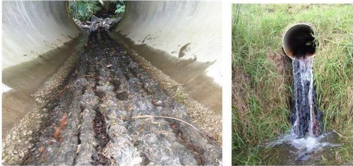
Figure 7. Mussel spat ropes installed in a perched culvert to facilitate upstream-migrating indigenous fish passage both into and through the culvert (in Lake Harihari) Photo: Bruno David).
