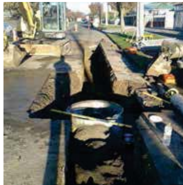
Below: Shoring protects Tasman Street stormwater work six metres below ground level.
