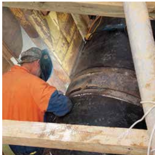
Installing a section of 900mm water main in Hargreaves Street, Wellington
