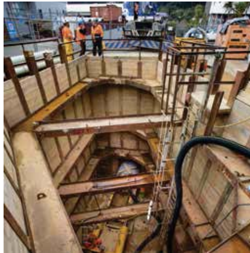
Below: Shoring protects Tasman Street stormwater work six metres below ground level.
