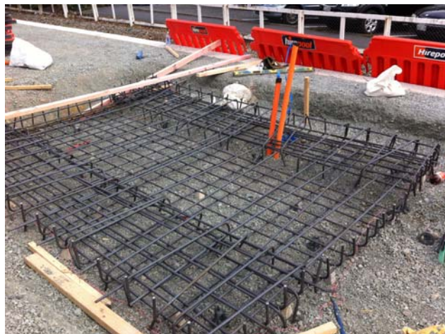
Fig. 2 Foundation cage being installed for new butterfly shelters
