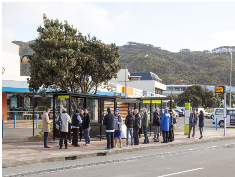
New bus shelter installed on Lyttelton Avenue (opposite Countdown Supermarket)
