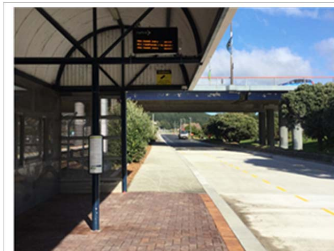
Porirua Station Road reconstruction, showing Kassel kerb installation and completed roadway
