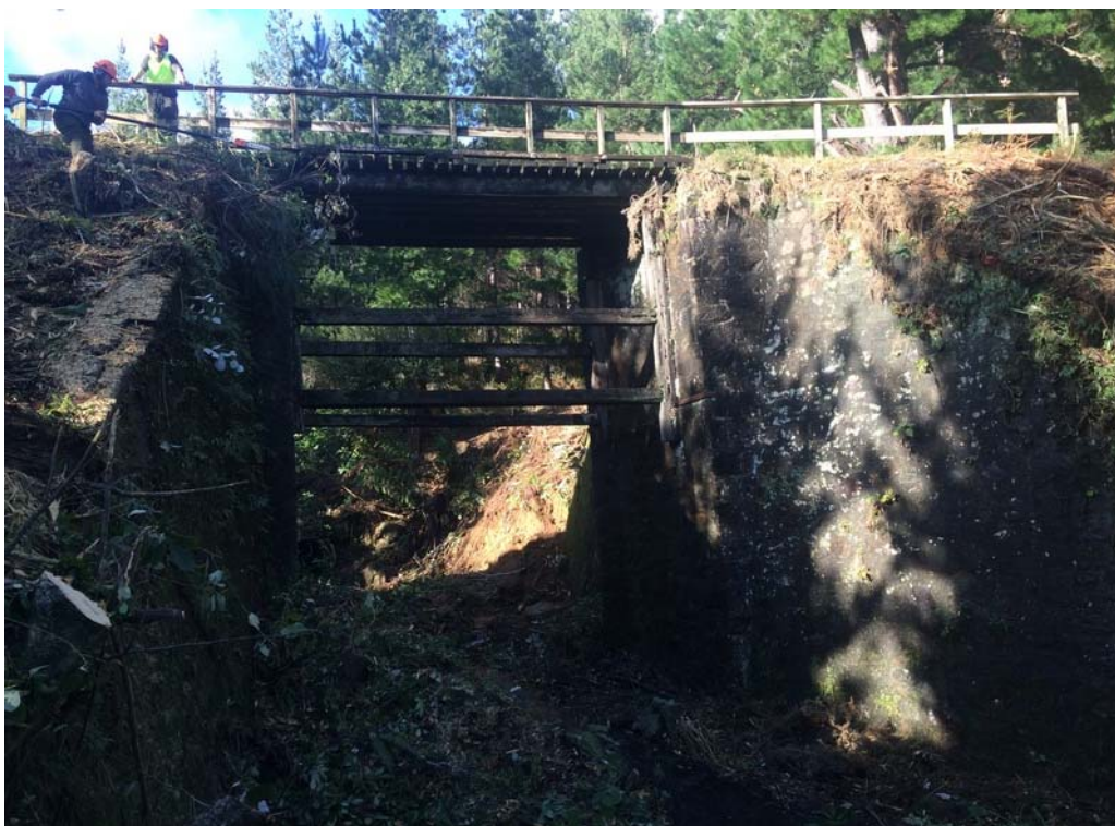
Historic stone bridge abutments and structure on Station Drive, Pakuratahi Forest.
