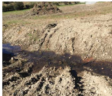
Unauthorised disturbance of stream bed from vehicle crossing
