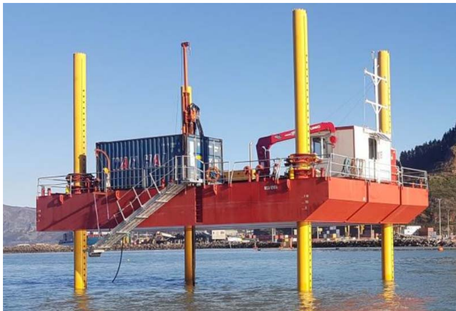
Photo: Heron construction
