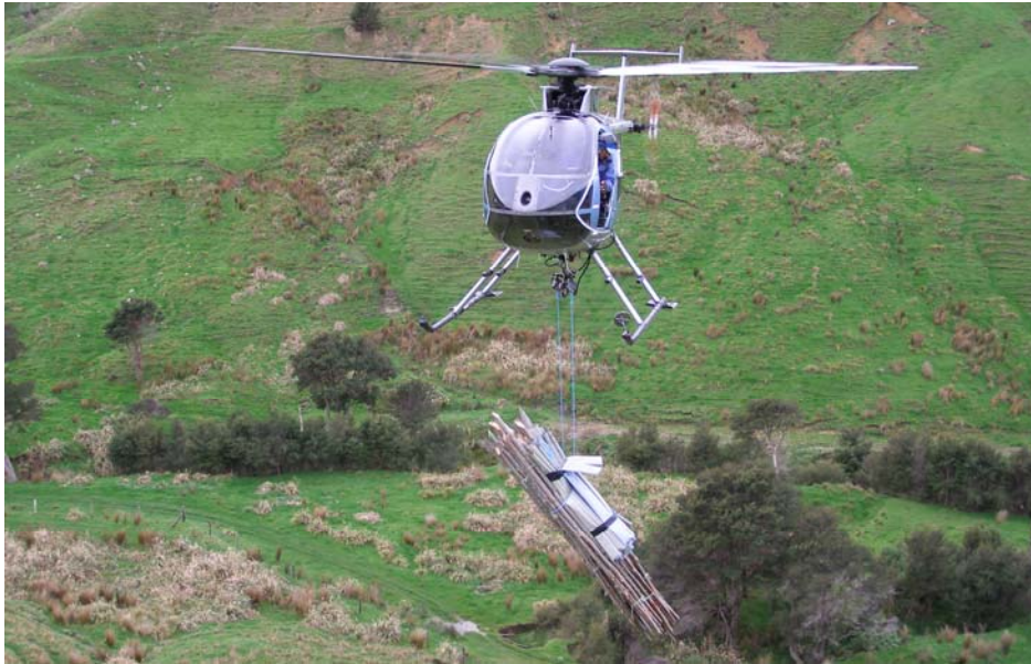
Pole delivery – Castlepoint Station
