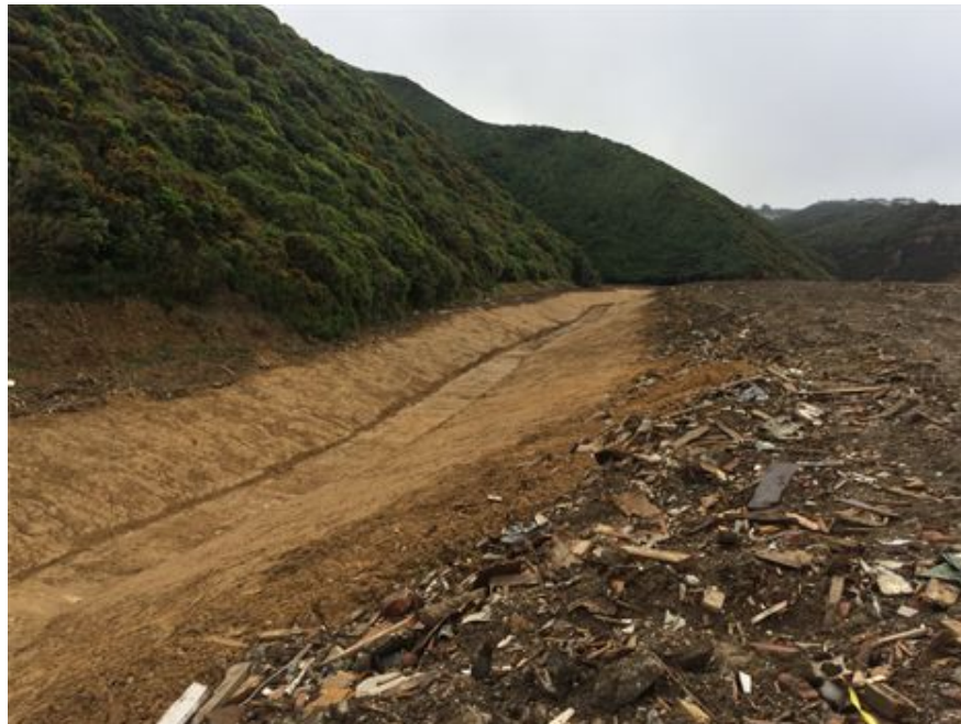
Photo of stormwater diversion channel from August site visit
