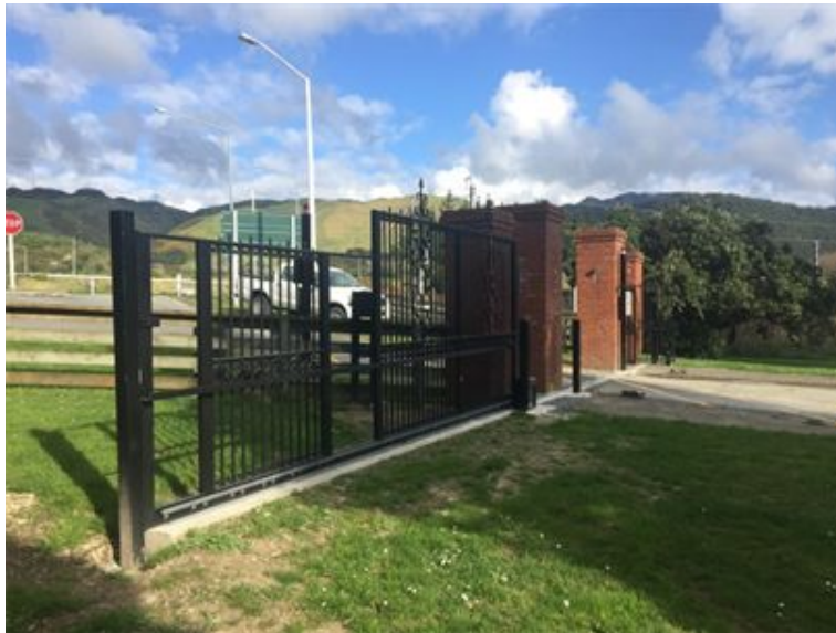
The new automated gate at Mackays entranceway to Queen Elizabeth Park
