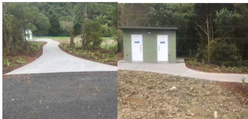
Landscaping around Dry Creek toilets begins
