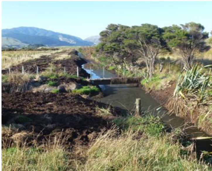
North Whareroa Stream following works. Note the still water; there is very little drop in height between Poplar Ave and Waterfall Stream further south.
