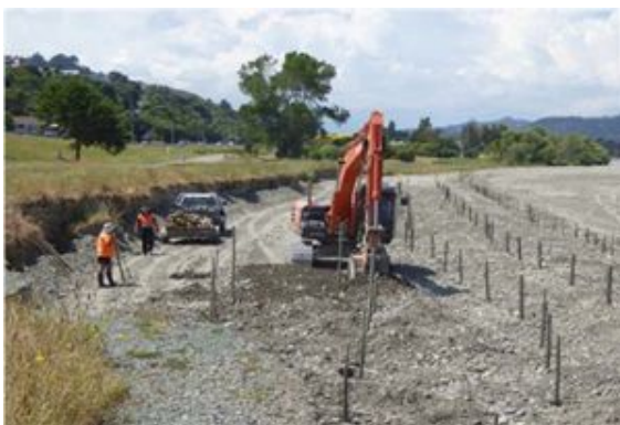
Hutt River Belmont edge protection works
