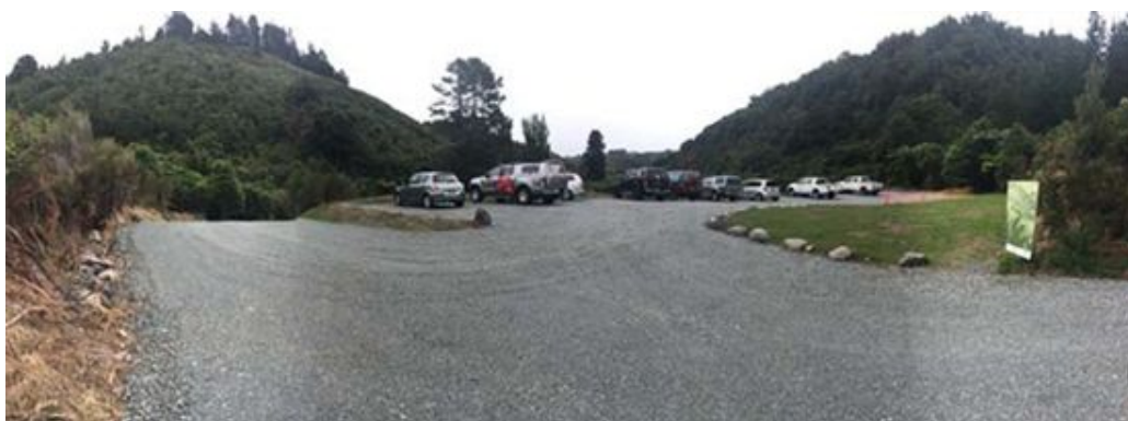
New carpark in former skid site; access to the forest at the right
