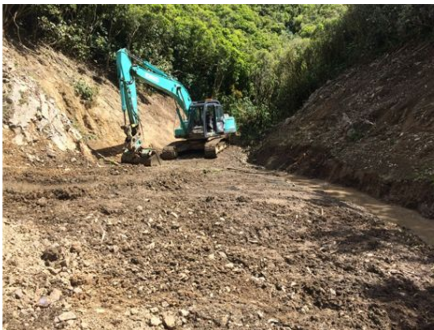
Finalising earthworks on eastern dam (November compliance inspection)
