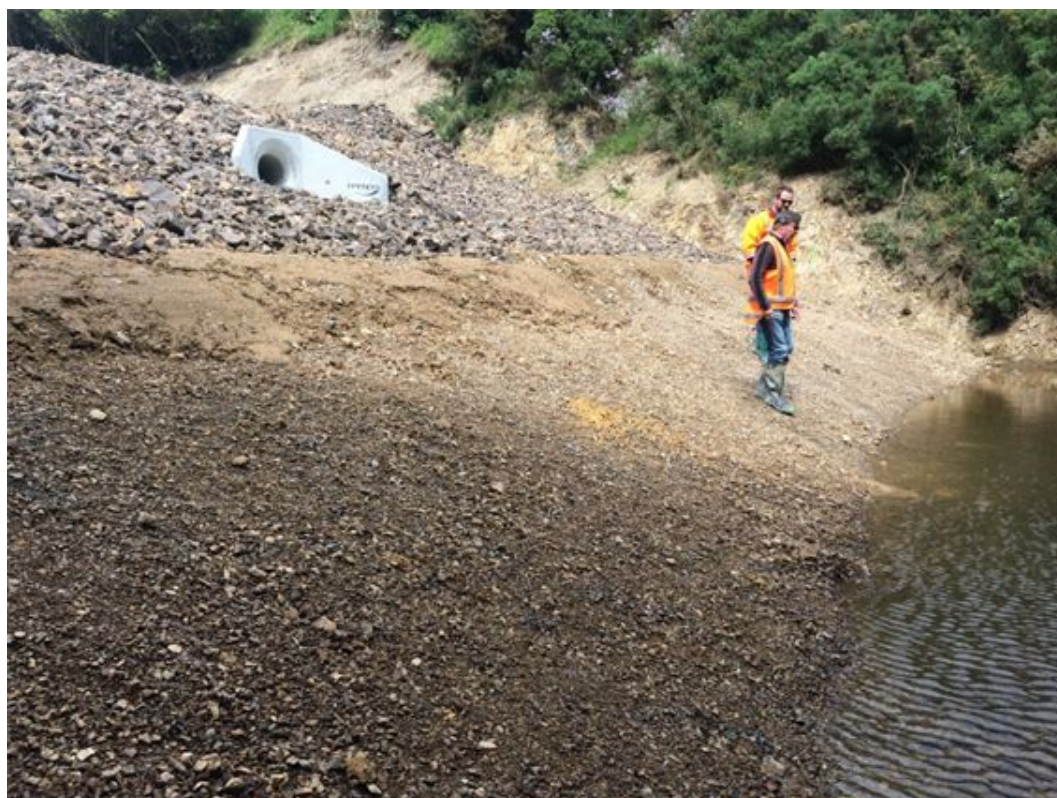
Western tributary Dam filling up (November compliance inspection)
