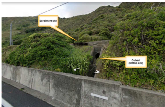
Figure 3 Culvert in relation to derailment location
