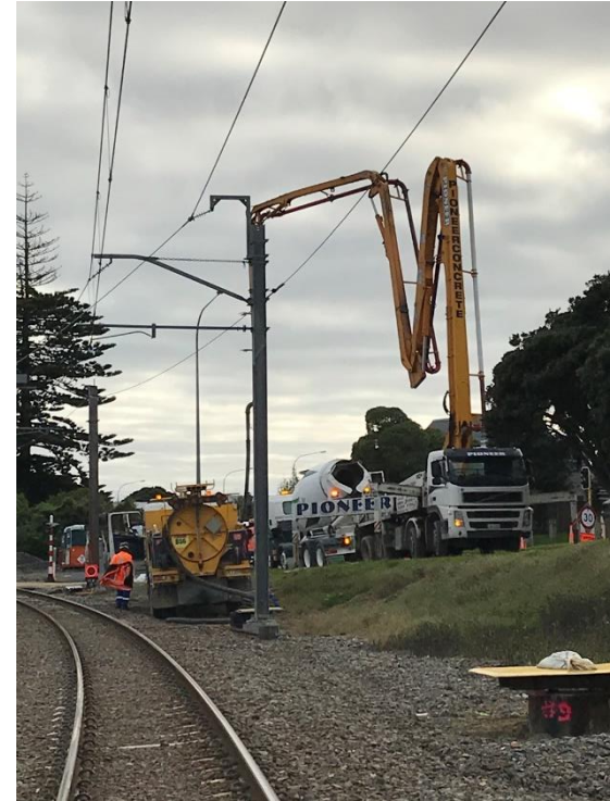
Concreting new pile at Plimmerton to allow OHLE to be realigned
