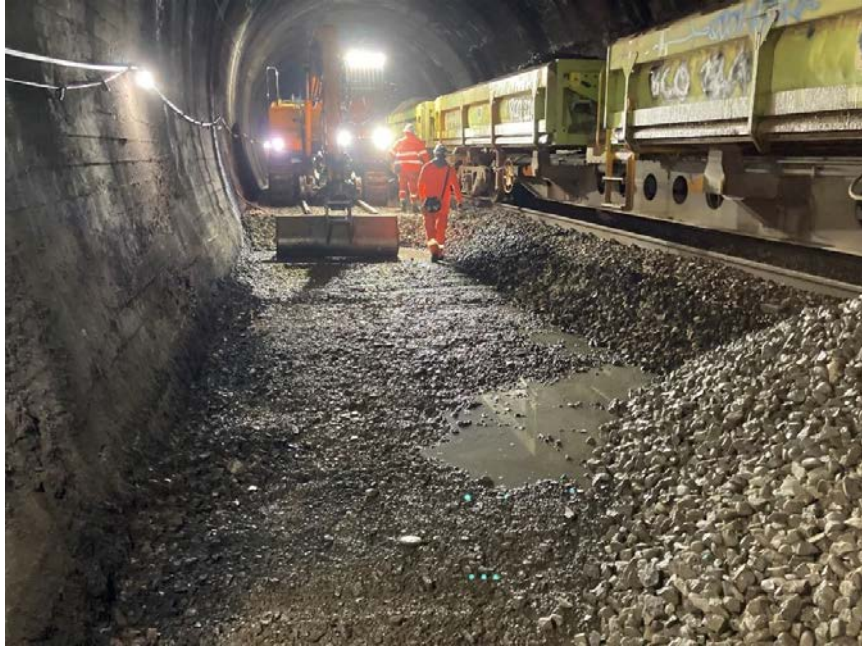
Tunnel 1 NIMT relay - Ballast removal using the YL ballast wagons (L) and relaying new track in panels for 100m section of Tunnel 1 Up Main on "Super Sunday" BOL on 18th July
