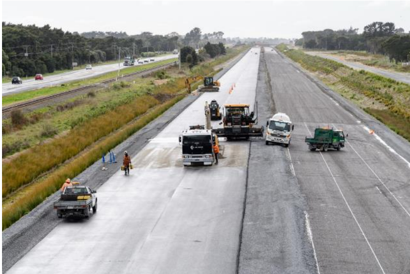
View from Te Horo overbridge – Bridge 8
