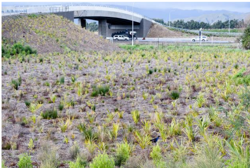
Wetland planting around Bridge 8
