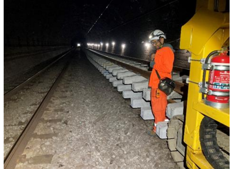
Tunnel 1 NIMT relay - Ballast removal using the YL ballast wagons (L) and relaying new track in panels for 100m section of Tunnel 1 Up Main on "Super Sunday" BOL on 18th July
