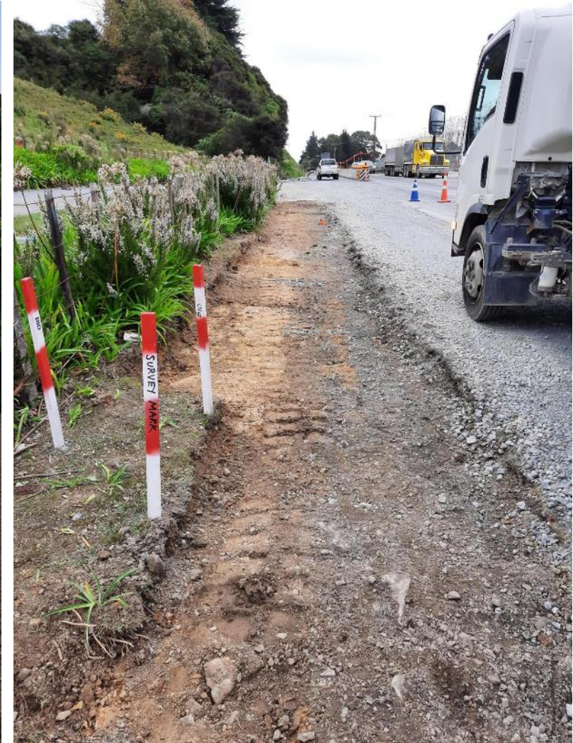
Surfacing preparation works
