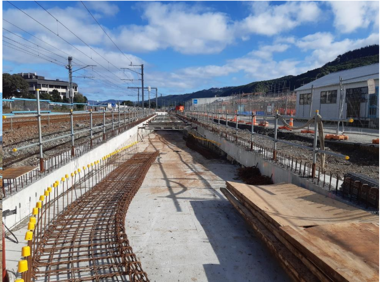
Ramp at Petone underpass taking shape
