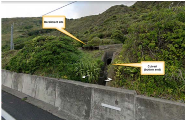
Figure 3 Culvert in relation to derailment location
