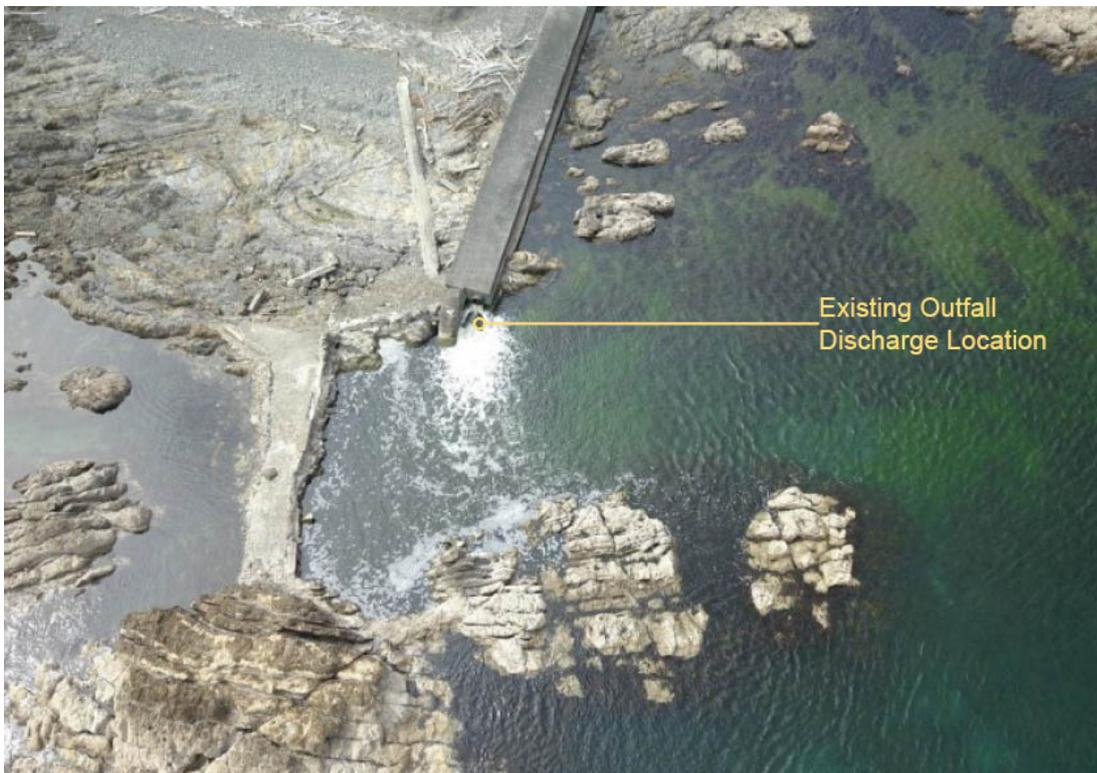
**Photograph 3:** Existing outfall at Rukutane Point showing pipe encased in concrete with concrete barrier to limit the immediate easterly flow of the discharge towards Titahi Bay. Photo from Figure 2: Aerial view of wastewater outfall at Rukutane Point, Memo from Dave Cameron 2 Dec 2019).
