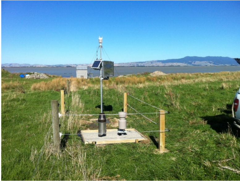
Figure 4.2: Recently installed GWRC met site on the western lake shore (an identical site was installed on the eastern shoreline); instrumentation includes tipping bucket and storage rain gauges, wind speed and direction, solar radiation and air temperature sensors
