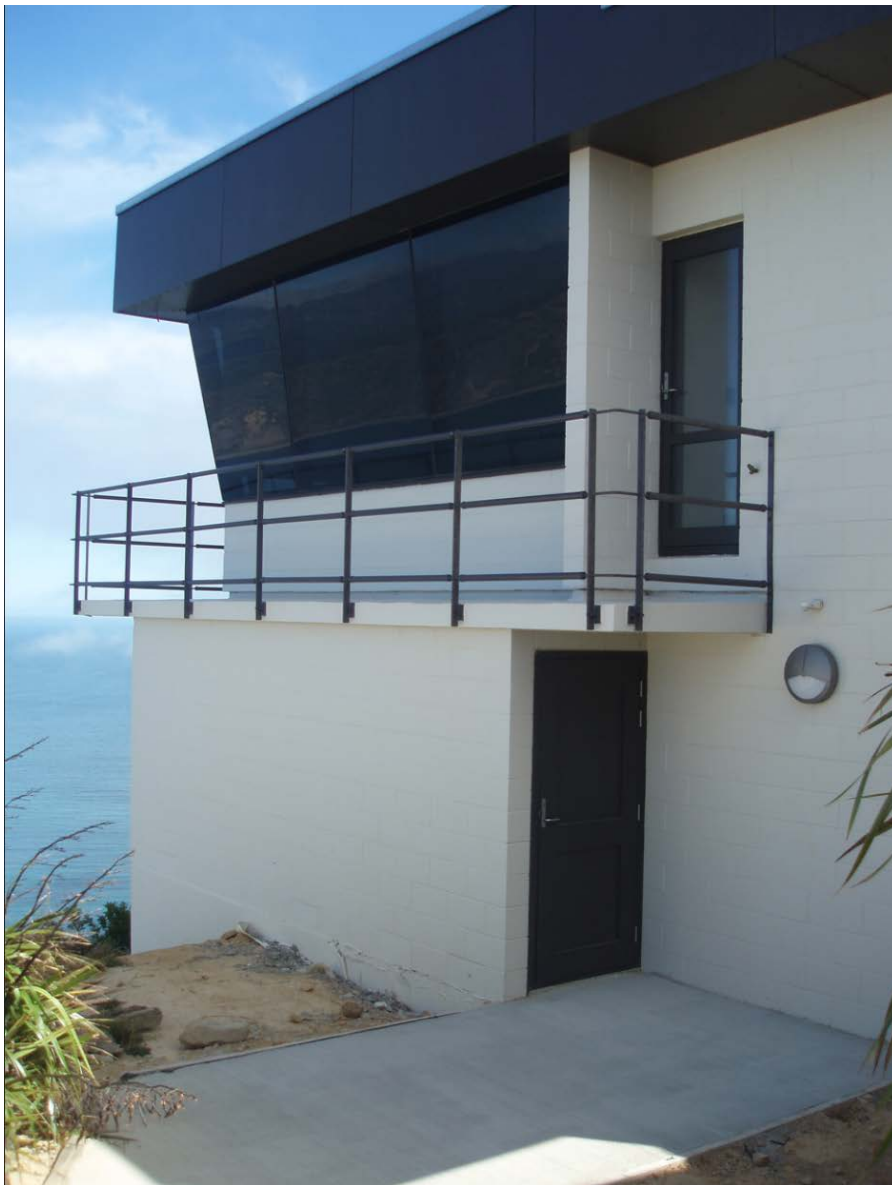
Figure 42 : Beacon Hill Signal Station
