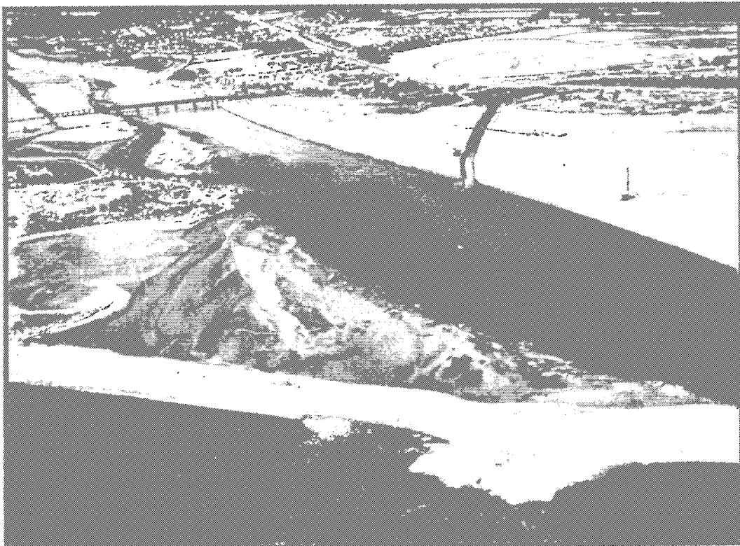
Plate 37: Shingle filling of the First Reclamation, c. 1934. Source: Alexander Turnbull Library, neg. F122250
