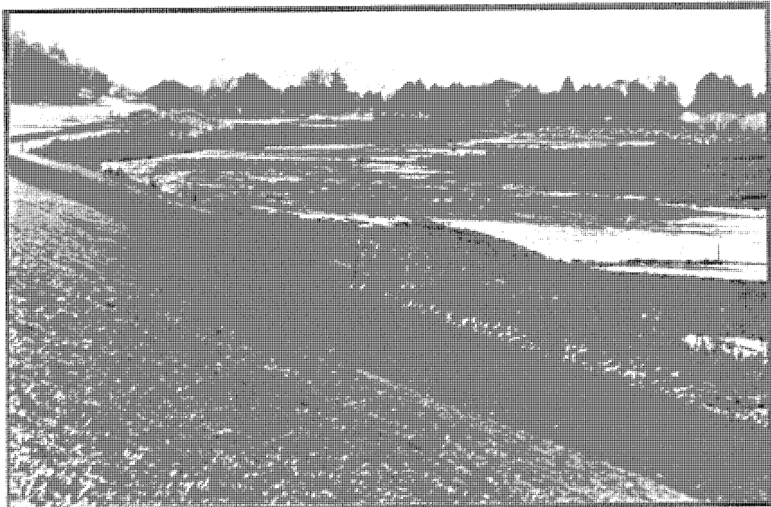
Plate 88: Newly Established Alignment, downstream Moonshine Bridge, 1986.
