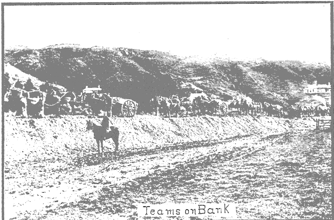
Plate 27: Construction of the first stopbanks - compaction. Source: Alexander Turnbull Library, York Studios, neg. F28346
