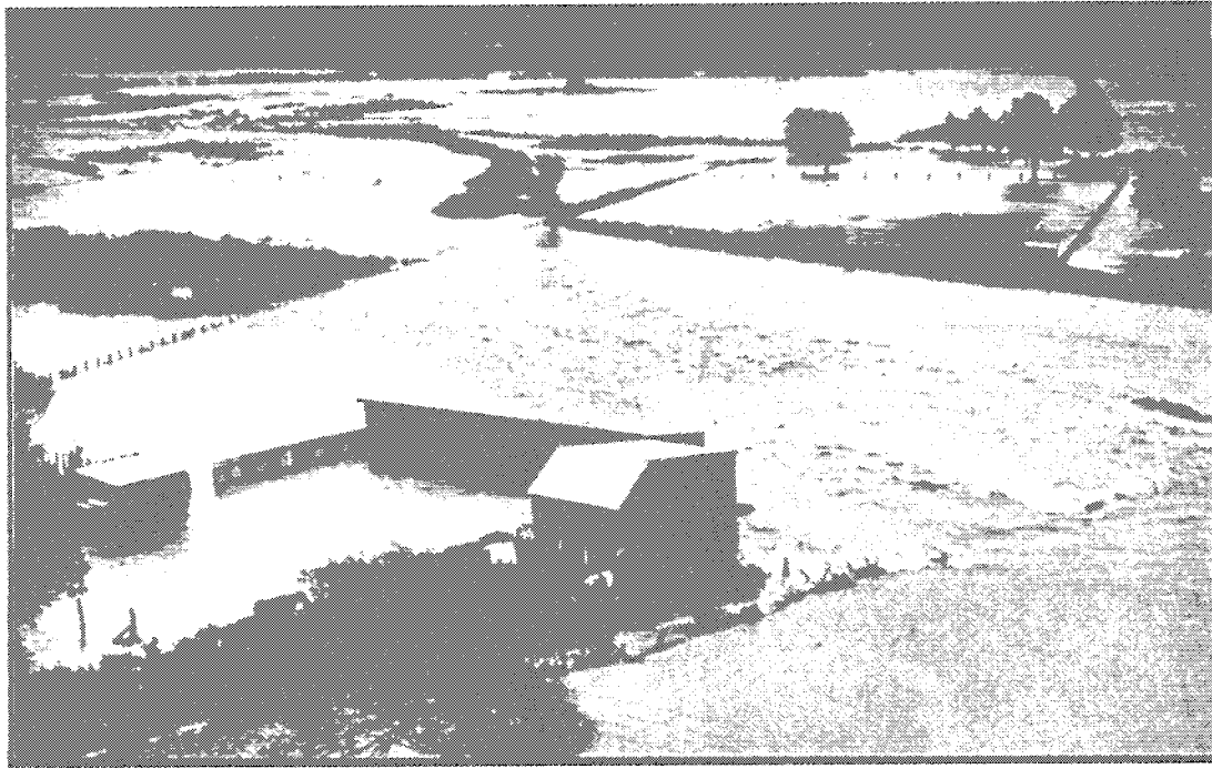
Plate 61: 1931 flood at Silverstream. Source: Treadwell.
