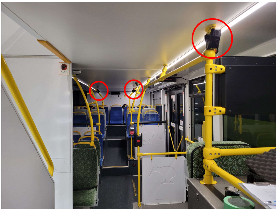
Figure 2. Example of the monitoring installation (red circles) in lower level of Bus 3701. Note on double decker buses the mid monitors were located back-to-back due to the location of the stairwell.
