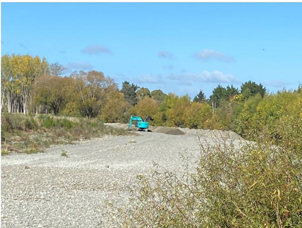
Figure 6: Site 12: River Road – Stage 2 – Temporary river diversion commenced
