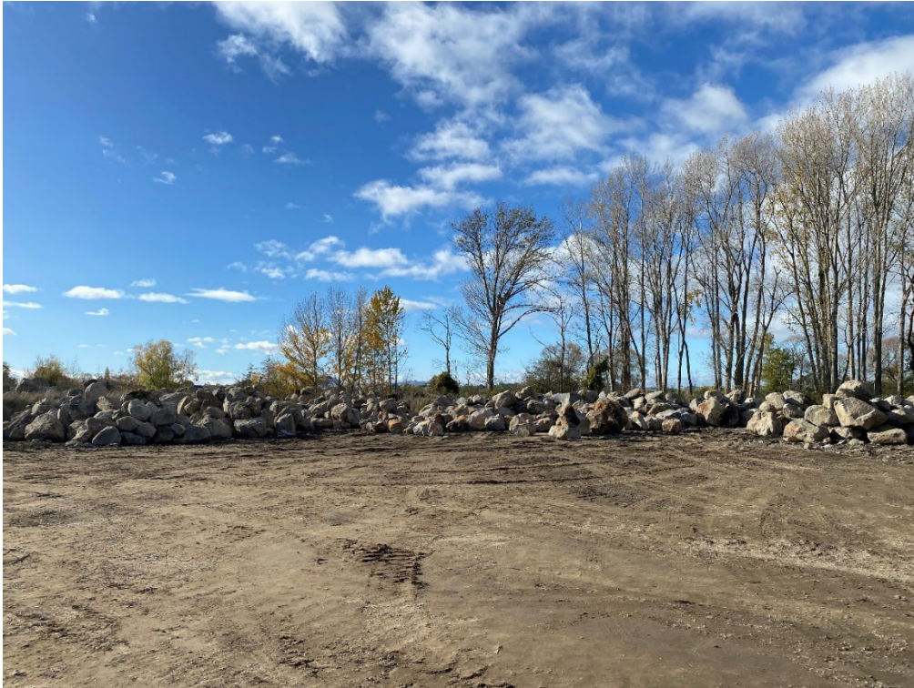
Figure 5: Site 12: River Road – Stage 2 – Rock supply
