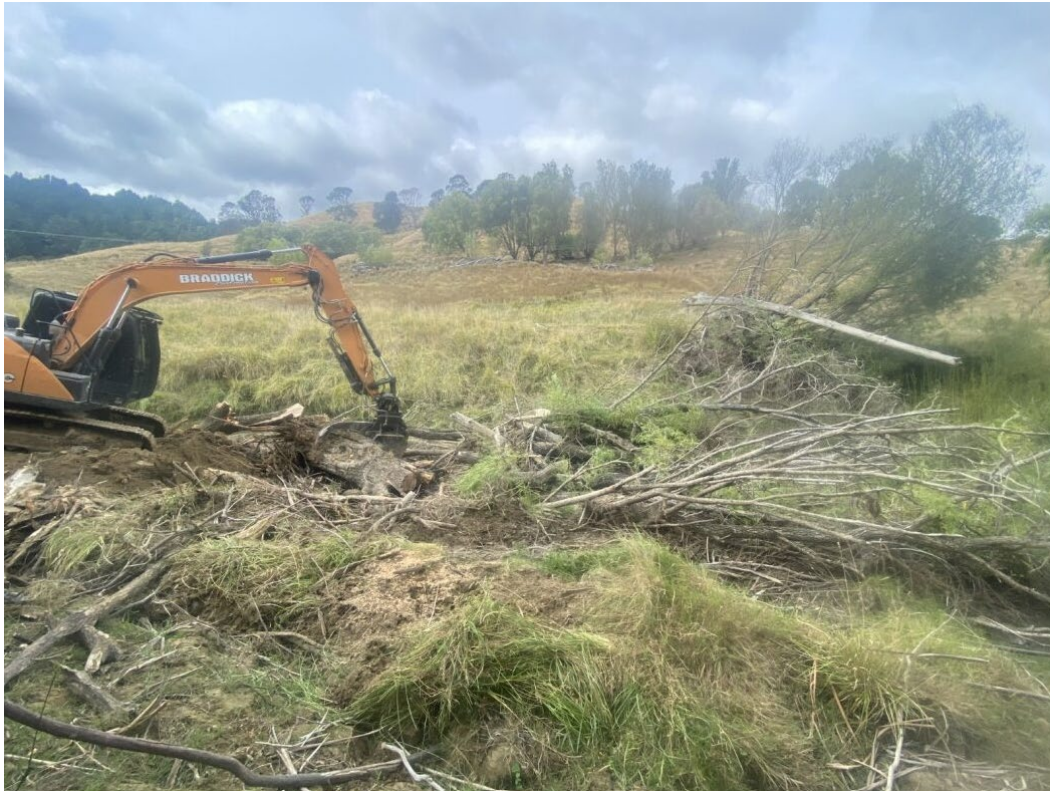
Figure 3: Whareama River – blockage removal commenced
