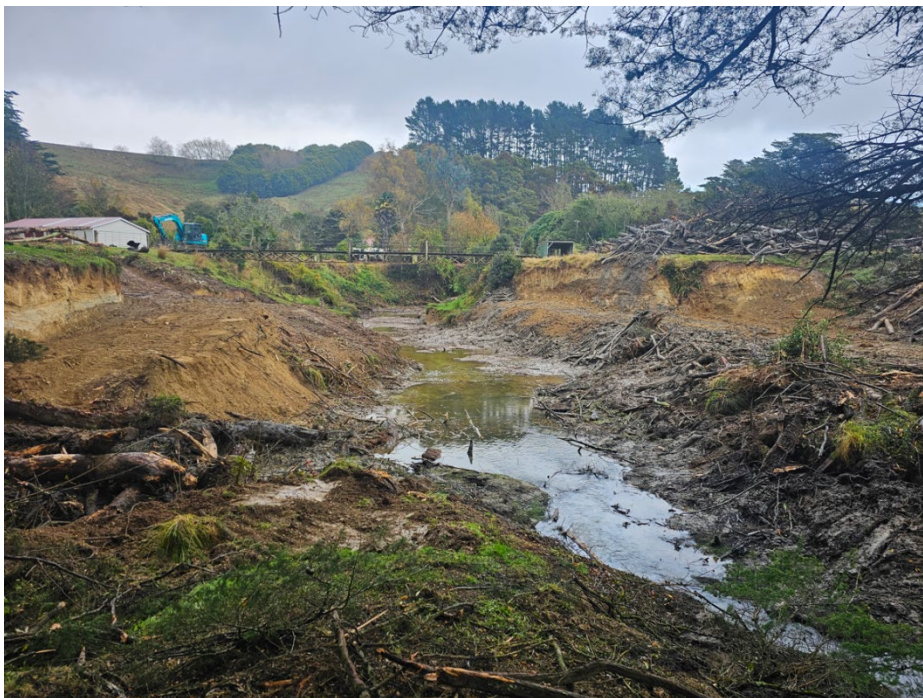
Figure 2: Kopuaranga River – post blockage removal
