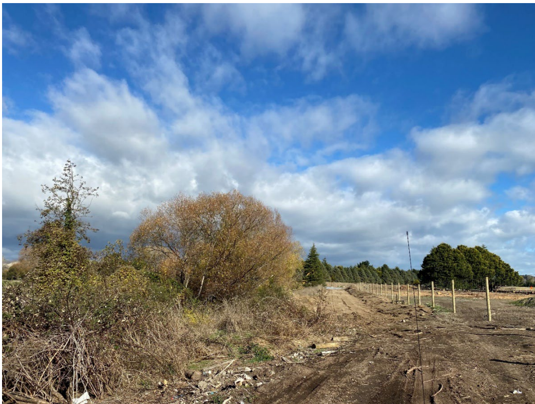
Figure 8: Site 12: River Road – Stage 2 – Haul Road commenced
