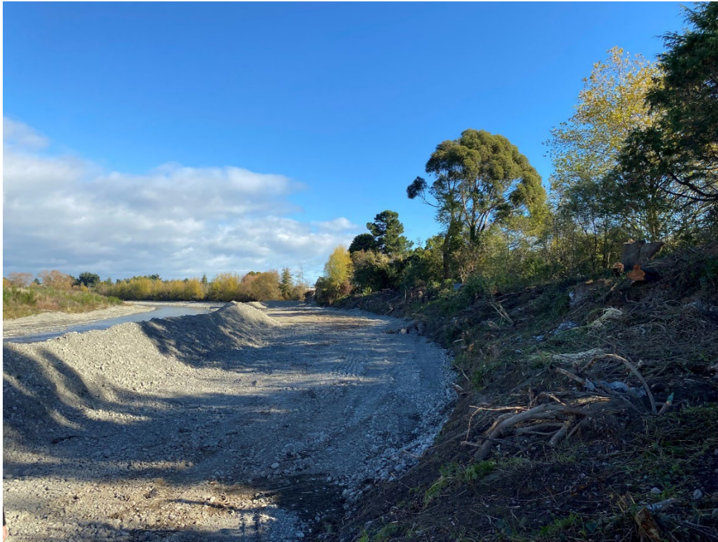
Figure 7: Site 12: River Road – Stage 2 – Temporary beach implemented
