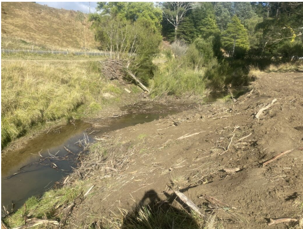
Figure 4: Whareama River – post blockage removal
