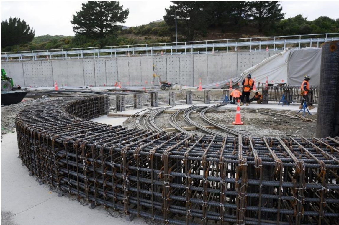
Figure 11: Porirua Wastewater Retention Tank Construction
