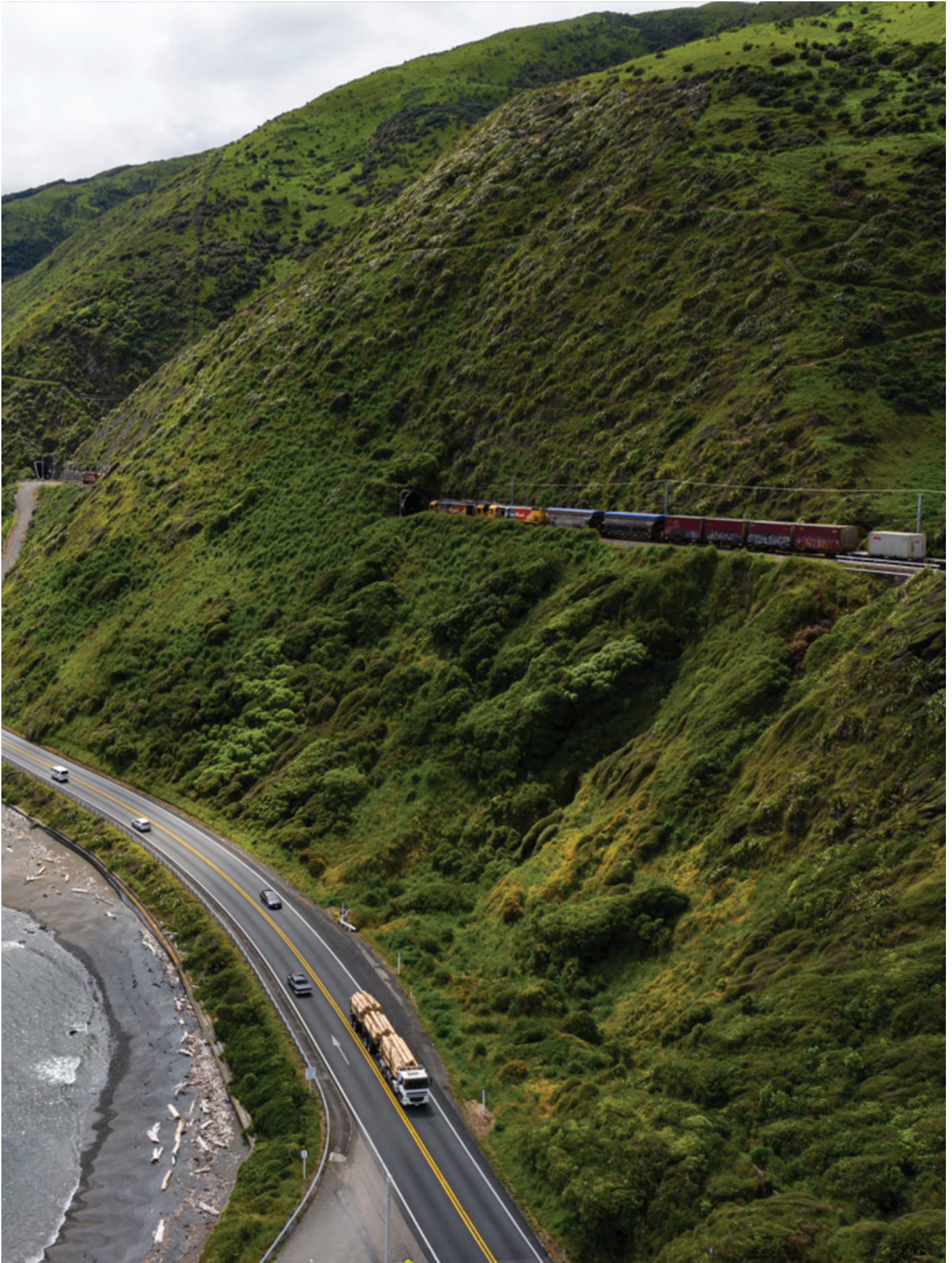
The Centennial Highway runs along the Kāpiti coastline while the Kāpiti rail line conveys KiwiRail freight and Metlink passenger services on the slope above.
