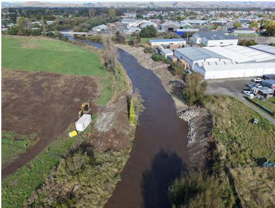
Photo 10: Site 4 – Waipoua Industrial Site (Akura Road) – five rock groynes and a 15m rock revetment completed
