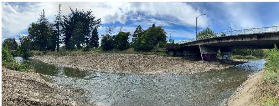
Photo 9: Site 3 – Waipoua SH2 Left Bank – 45m rock revetment completed
