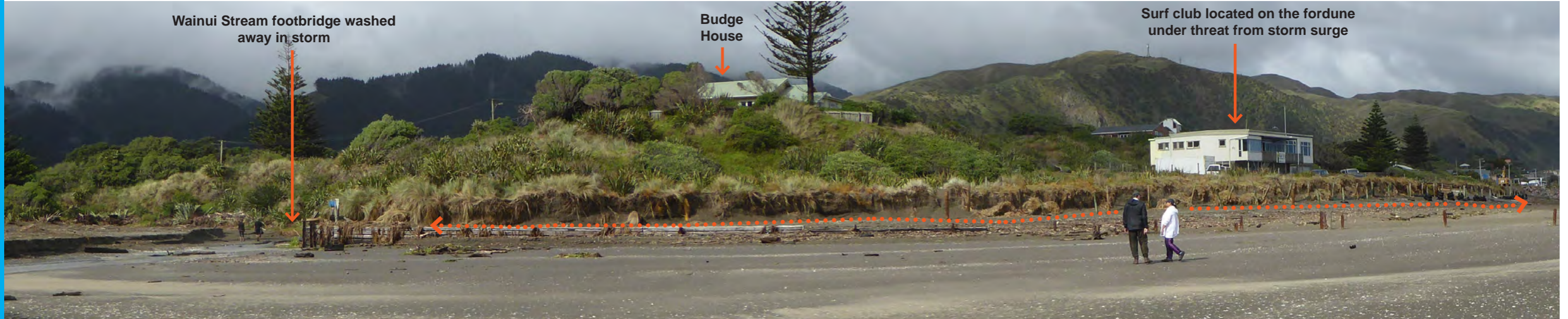
Erosion at toe of foredune below Budge House and surf club
