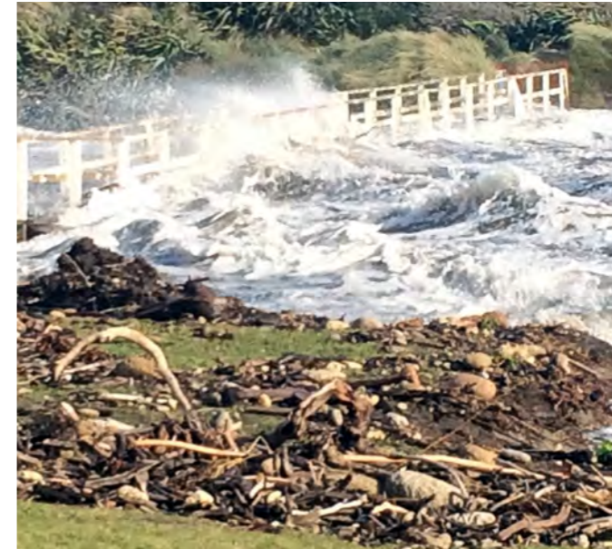
Footbridge during storm early 2018
