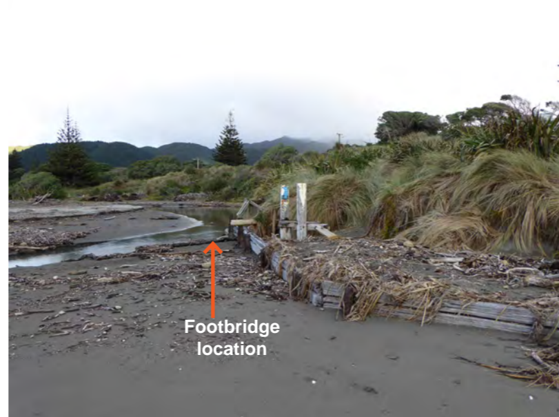
Footbridge across Wainui Stream washed away
