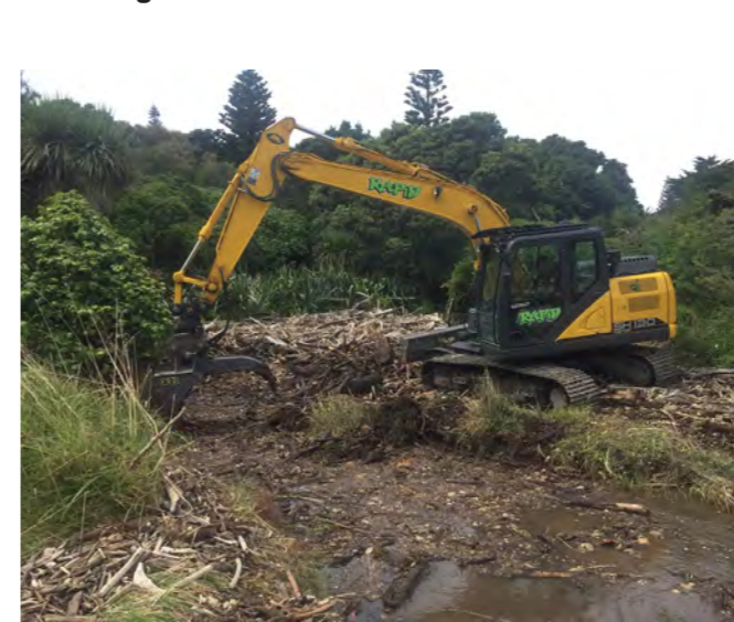
Clearing debris from the stream after storm 2018
